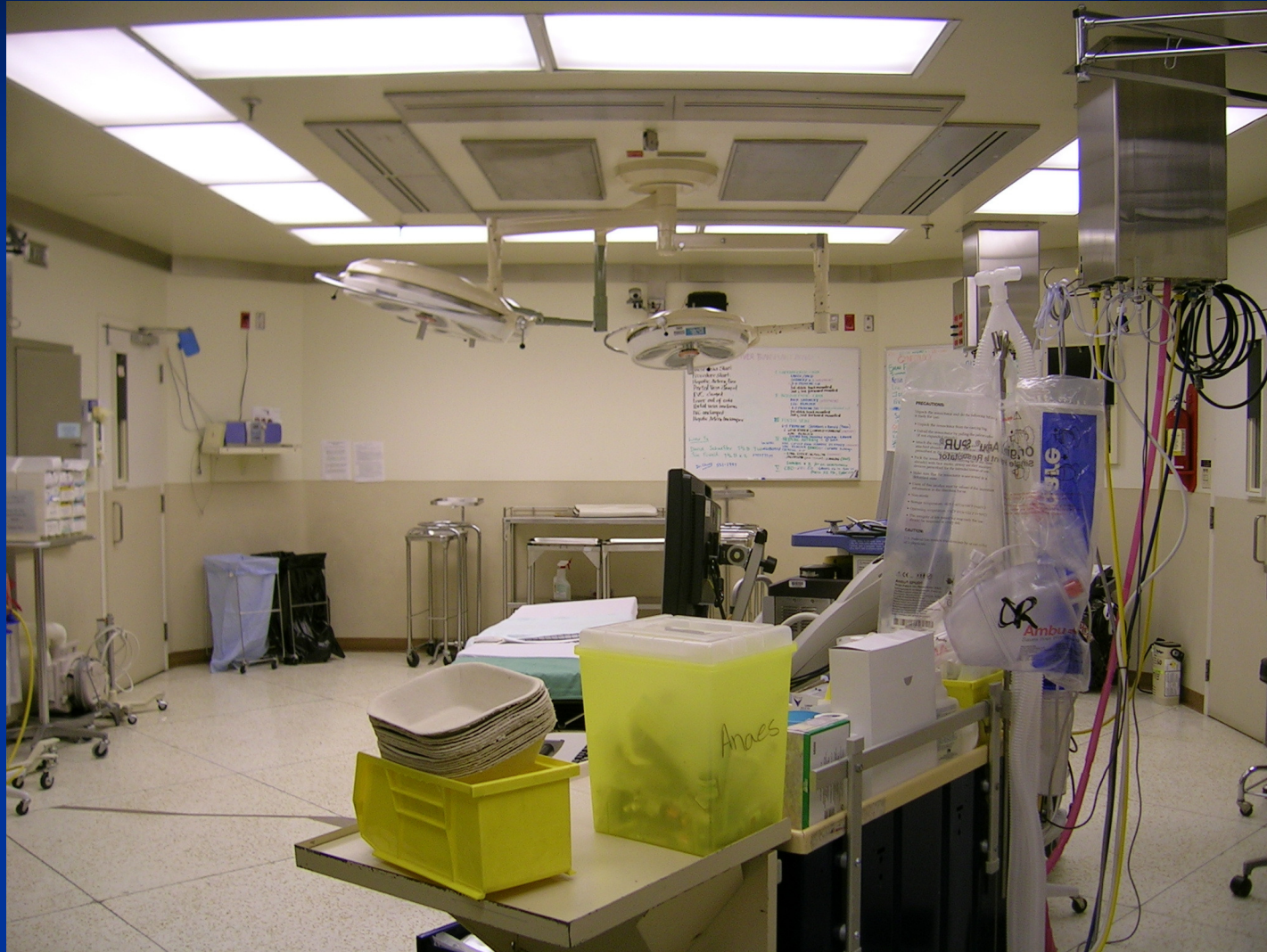
Vancouver General Hospital: JP North OR9 Laminar Core with Perimeter Air Curtain
